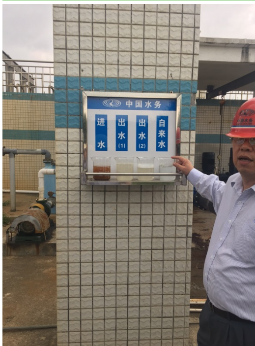
Exhibit 9: Site manager shows water treatment by stage
